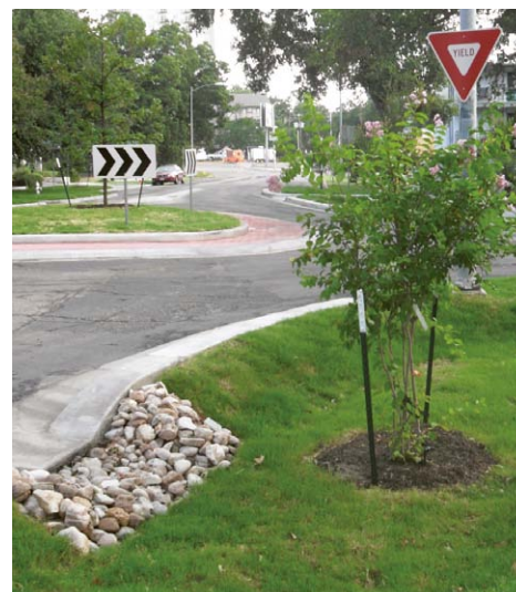
Curb-cut swale in Austin, an example of low-impact stormwater management.
